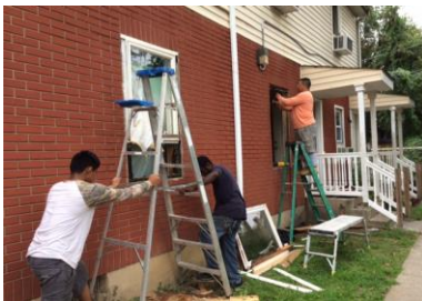
Installing New Windows
