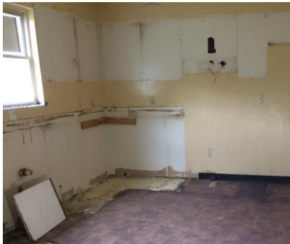
Kitchen Before Rehab – Sad and Empty
